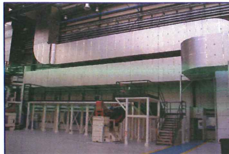
ALP System ductwork installed in Alenia Aeronautica's new Factory in Grottaglie
